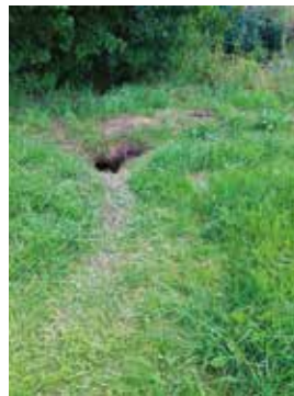
Trail to landside collapsed burrow entrance
