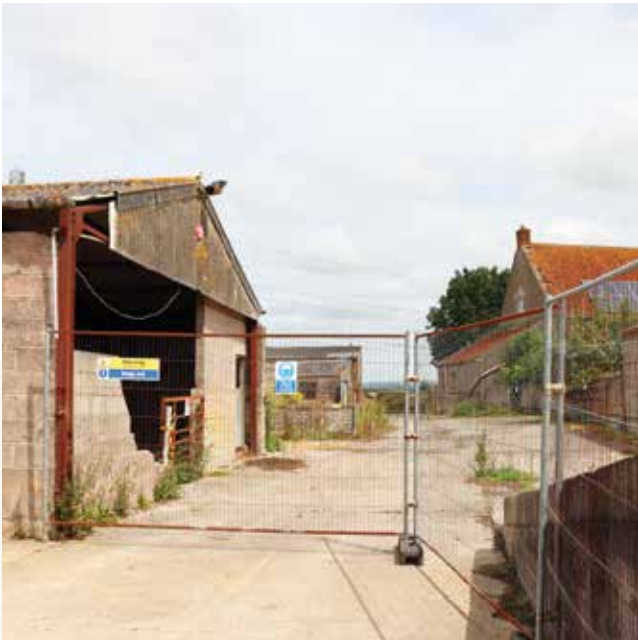
Original buildings on site
