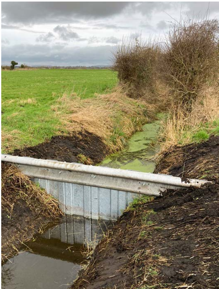
SHEET PILE DAM IN DITCH TO RAISE THE WATER LEVEL
